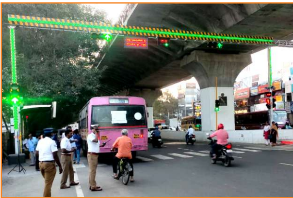
PELICAN SIGNAL (PEDESTRIAN CROSSING)
